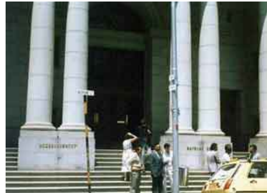
Supreme Court Building, Cape Town
